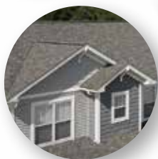
Roofing and Ventilation
