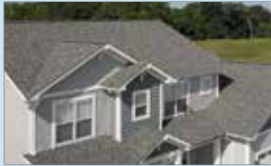
Roofing and Ventilation
