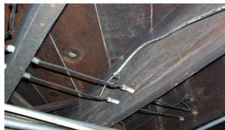
Fig. 4 – K&T wiring through joists
