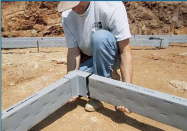
Lineal sections, couplings and corners ensure precise form set-up — allowing for a very flat and level footing.
