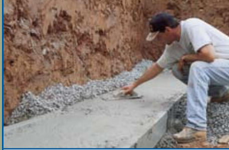
Form-A-Drain is both the footing form and the foundation drainage system, allowing you to accomplish two jobs at the same time — saving time...and money.
