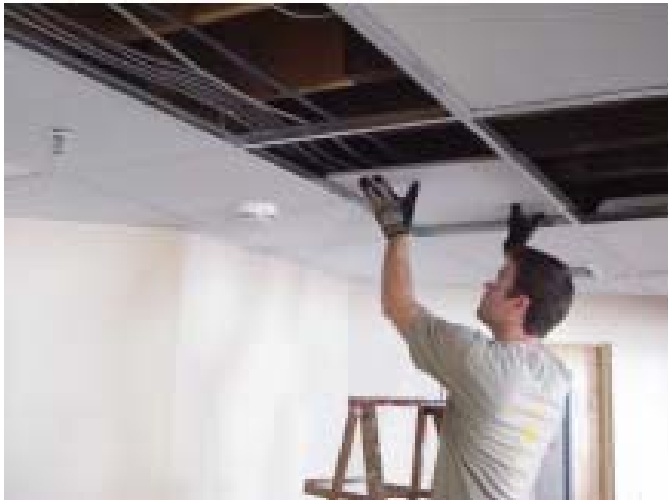
Figure 2: Example Ceiling Panel Installation
