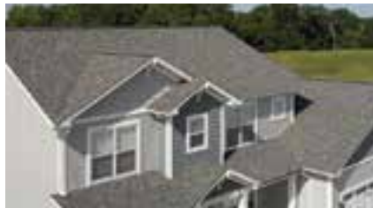
ROOFING AND VENTILATION
