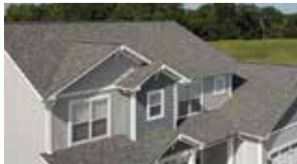
ROOFING AND VENTILATION
