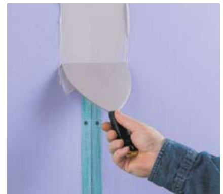
Self-adhesive tape saves time by eliminating the need for a pre-bedding coat.
