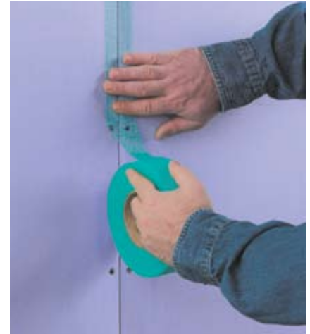
Self-adhesive tape saves time by eliminating the need for a pre-bedding coat.
