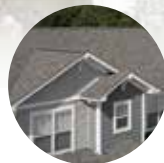
Roofing and Ventilation
