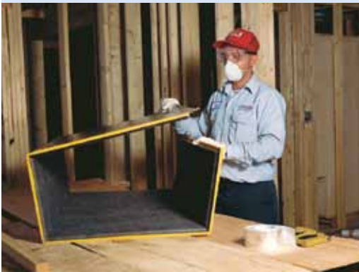
Fiber glass duct board is fabricated into a rectangular section of a fiber glass duct.
