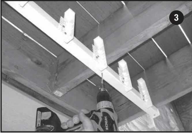
**Step 4:** Level and shim grid bars as needed. If using a gutter system you may want to install gutter before installing last grid bar.
