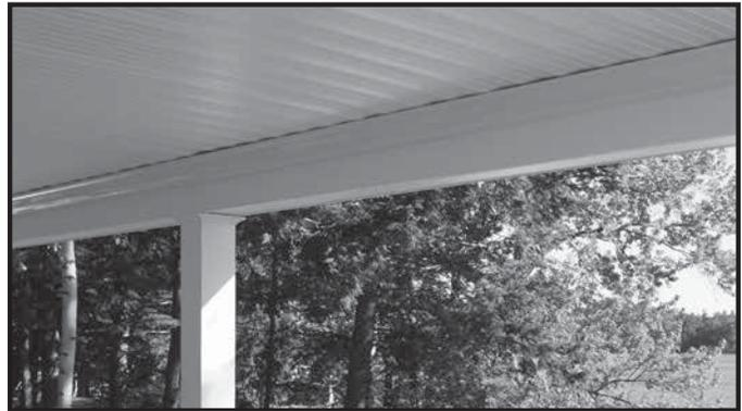
**NOTE: Locking the panels together creates a tight lock. Panels will not easily slide on each other. Be sure to line up panel ends before zipping over the hooks of the previous panel.**
