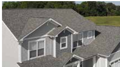
ROOFING AND VENTILATION
