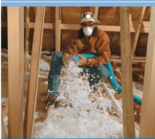
Blown-in fiber glass can be installed with pneumatic devices to meet almost any R-Value requirement.
