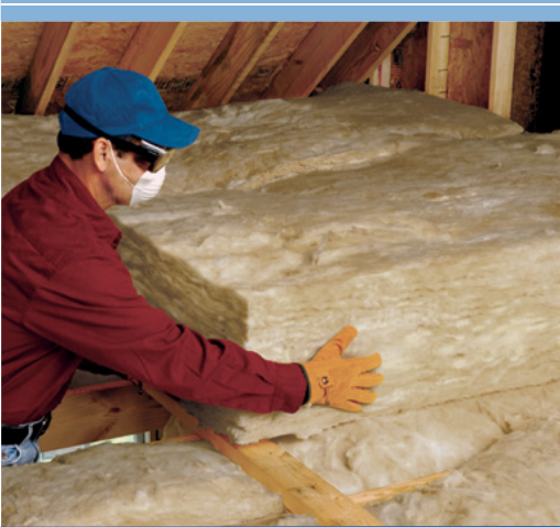
Application of fiber glass batts in an attic.
