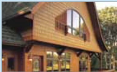
Fiber Cement Siding
