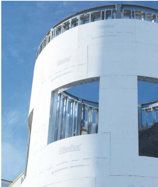
CertainTeed's GlasRoc ® High Performance Sheathing provides enhanced dimensional stability, yet it is flexible enough to bend to curved surfaces, like the towers at The Avenue at Westchase.
