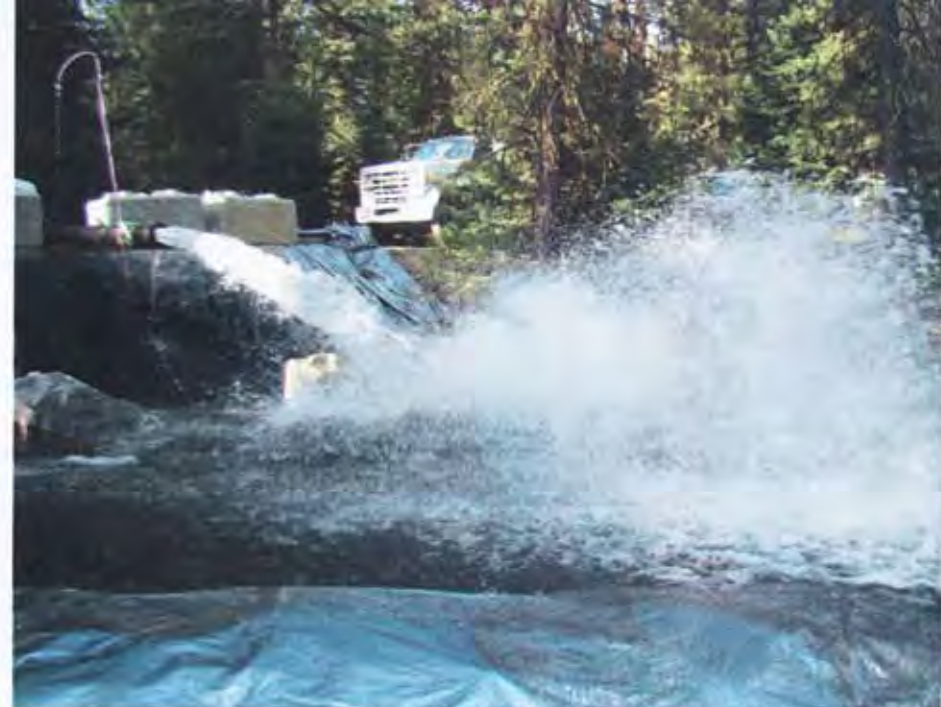
ACHIEVING 3,300 GPM AT TAMARACK'S #10 WELL.
