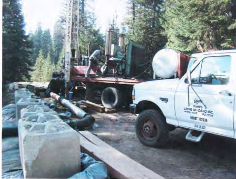
ON SITE DURING THE WELL DEVELOPMENT PHASE.
