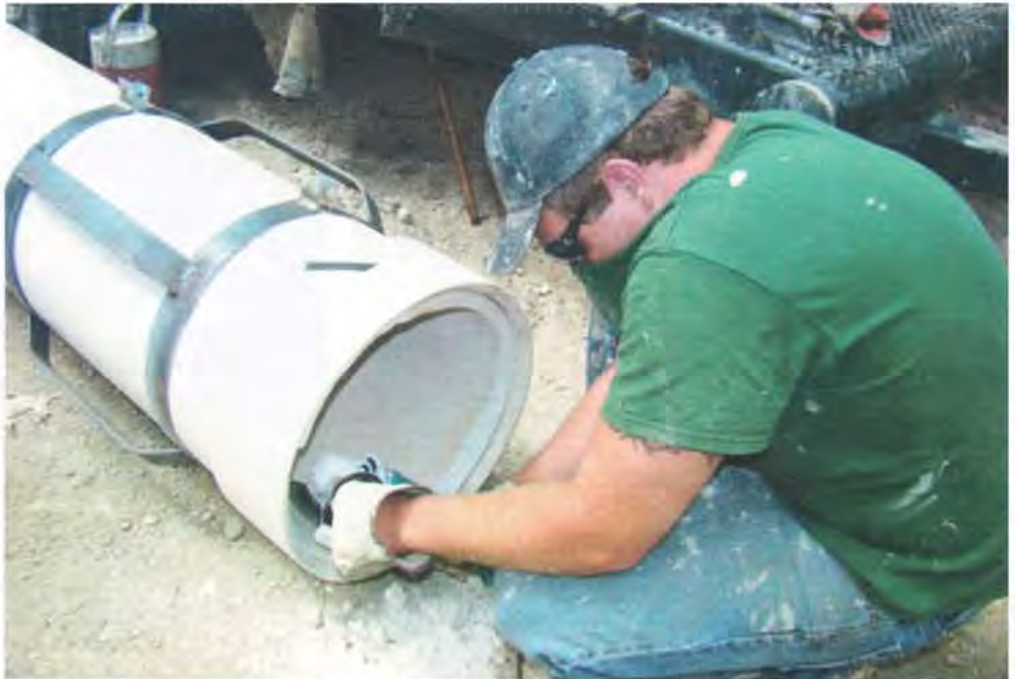
PREPPING FOR INSTALLATION.
