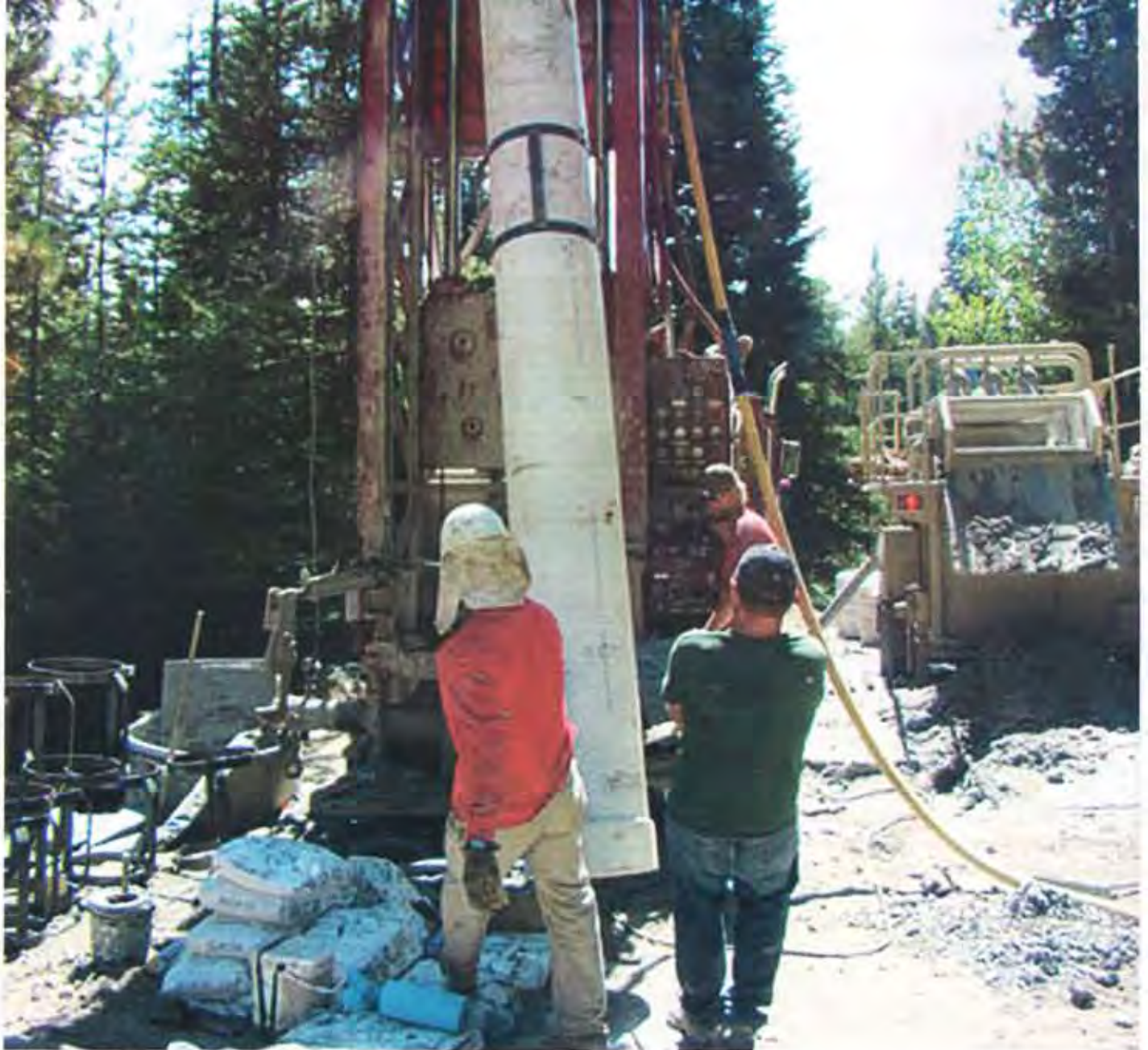
INSTALLING THE PVC CASING.
