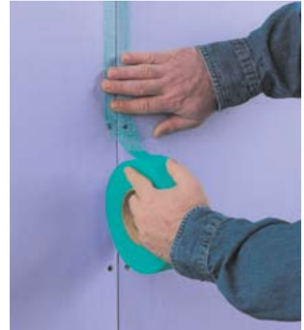
Self-adhesive tape saves time by eliminating the need for a pre-bedding coat.
