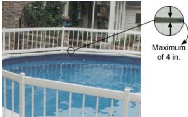
The fence is on top of the pool
